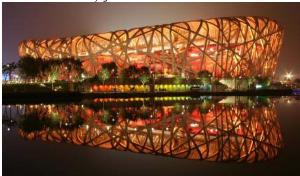
Photo 1. The National Stadium in Beijing 'Bird's Nest'
